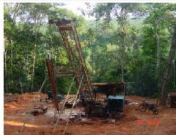
Photo 4: Drilling rig in operation at Serra Guemada Target.
