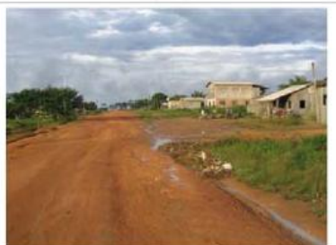
Photo 9: Transamazônica road Km 180 crossing bridge (gas station, market, lodging, telephone).
