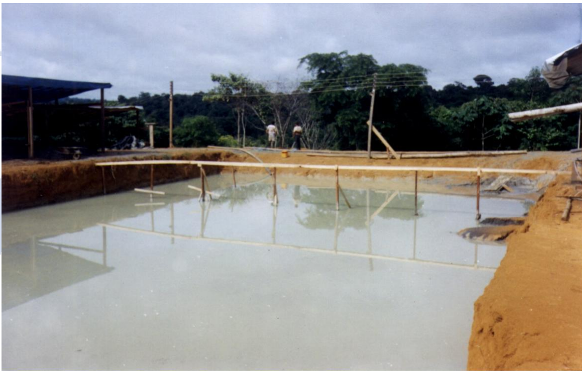
Figure 14: pool of solids settling
