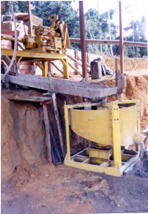
Figure 19: ourocone placed in series with industrial mill
